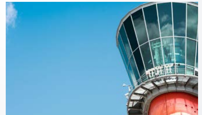
Cover image: Heathrow Airport control tower © Heathrow Airport
